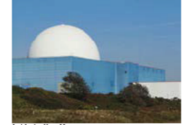
Back Facades of Turbine Halls
