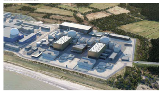
An aerial view of Sellafield C Operational Site
