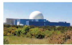
Current site of Sizewell C's dome and associated buildings.
